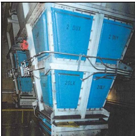
This photograph shows the FRP Heating Panel installations on the main Truck Dumper Hoppers at the Colver Power Project located in Cambria County, PA.
