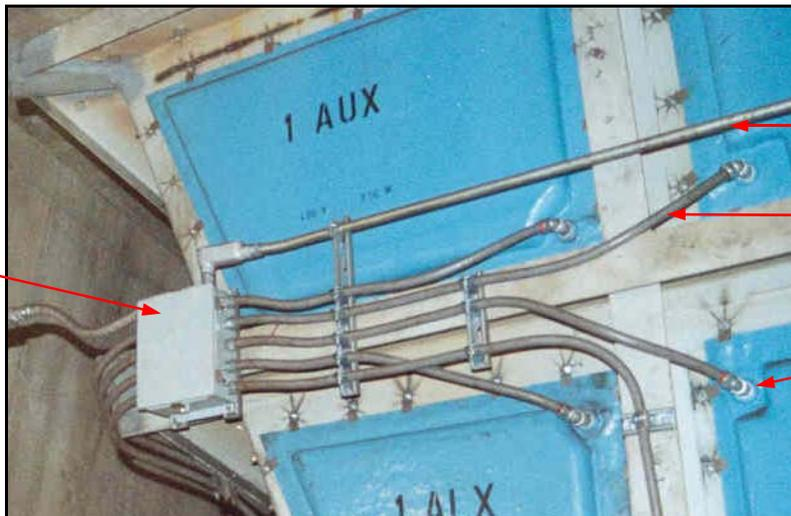
Local mounted junction box to accommodate the connection of all of the heating panels installed on two sides of a hopper
